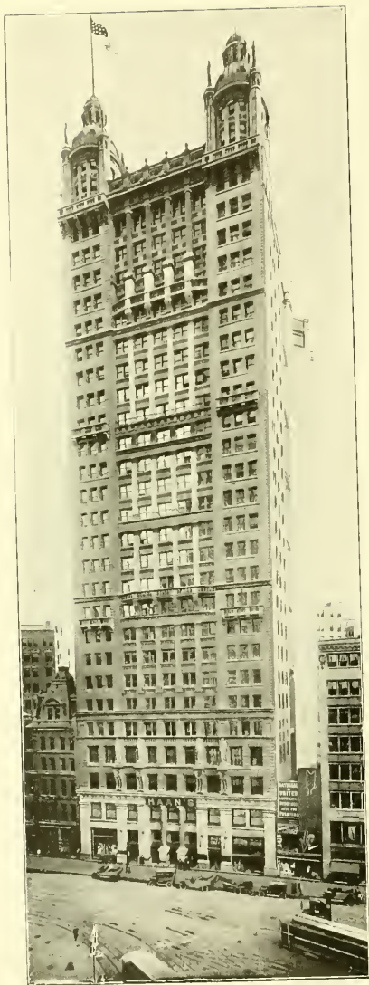
PARK ROW BUILDING —Located at the head of Park Row, opposite the General Post Office adjoining Ann St. It rises to a height of 29 stories including tower, 381 feet high. It is built entirely of lime stone and has the distinction of being the first skyscraper in New York, being ready for occupancy in October, 1889. Total cost, $3,500,000.
